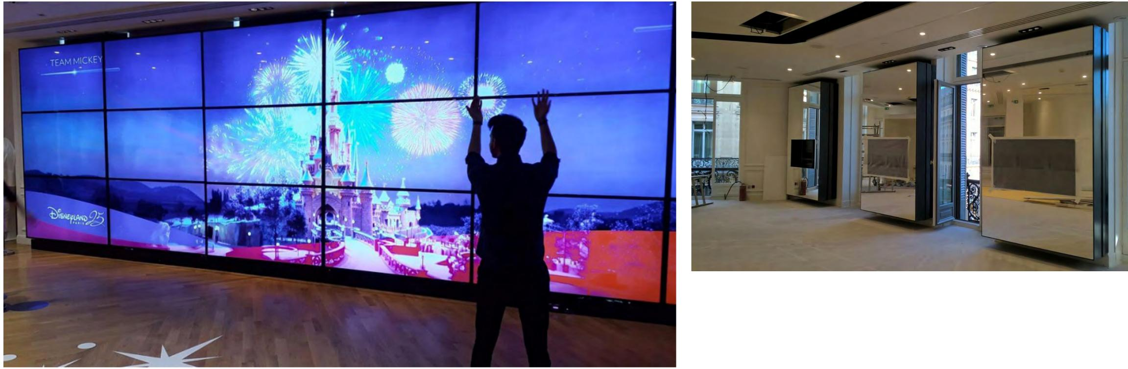
998 x 282 cm LED-LCD wall with 18 75-inch monitors at ORANGE - event space in central Paris. LED wall management via RTI control, Modulo-Pi station and Extron XTP grid.
