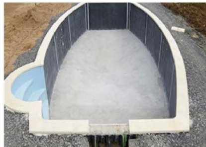
2. Liner (PVC) Interior Finishing
