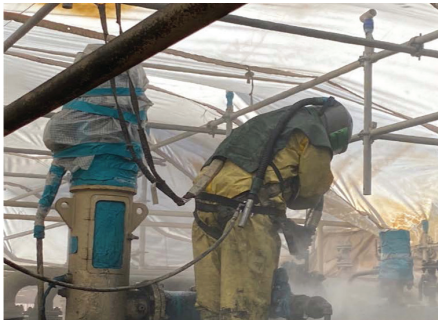
Fig. 4: The contractors used wet abrasive blast-cleaning to prepare the steel tanks.
