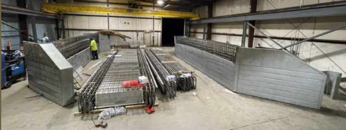
1 Pre-fabricated components manufactured in controlled environment
