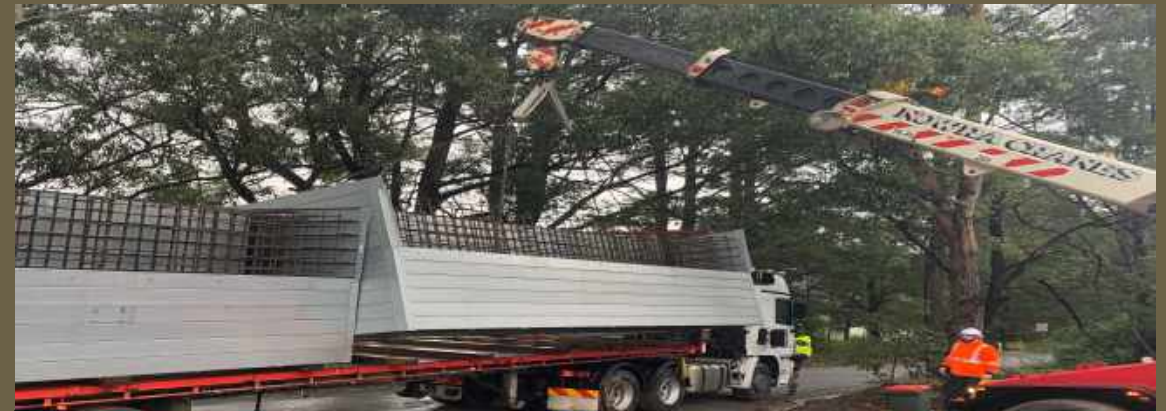
4 And handled by small cranes or excavators
