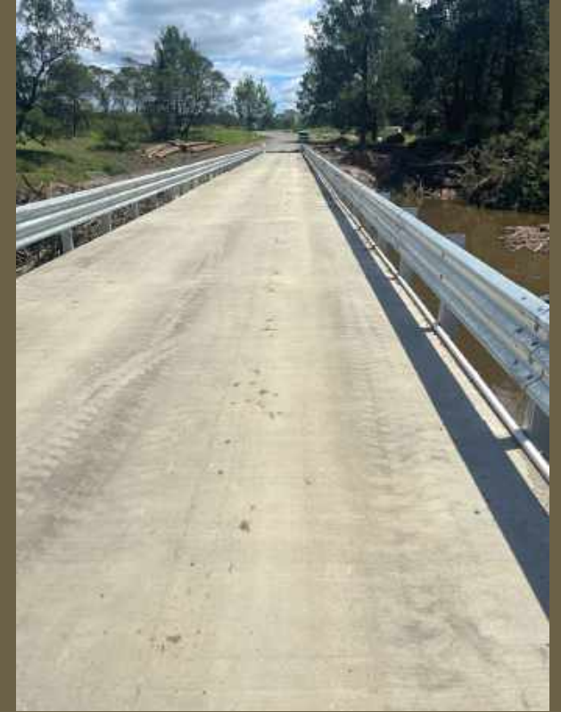
After removing debris
