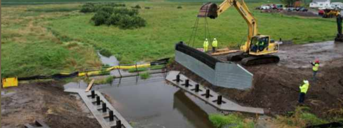
1 Abutment placed into position and filled with concrete
