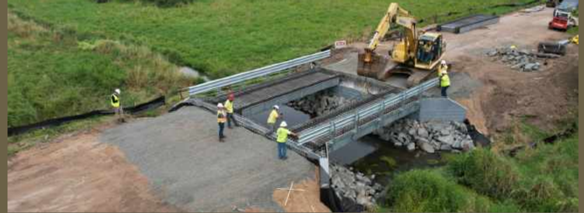
2 Decks placed and tied together to create one large mass
