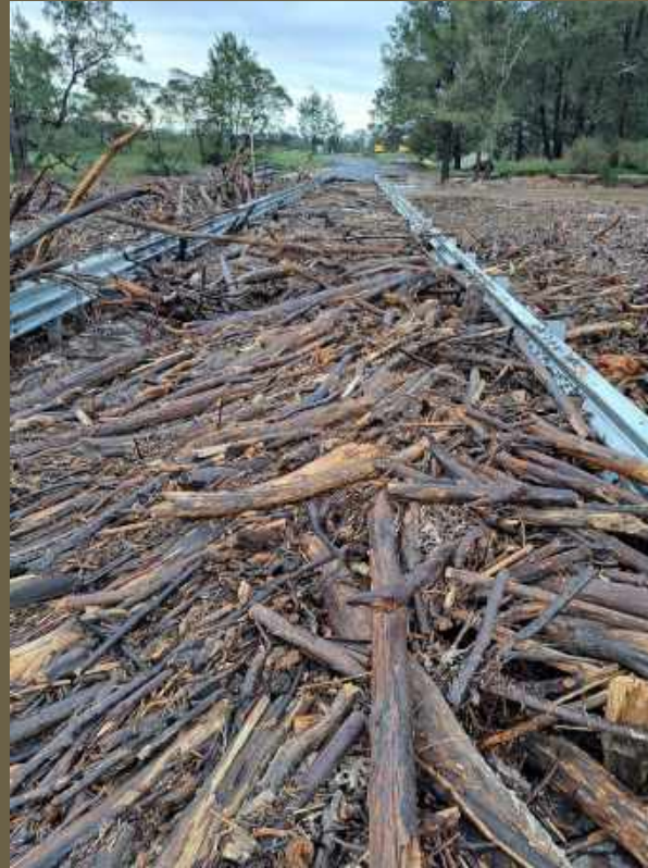
After flooding event
