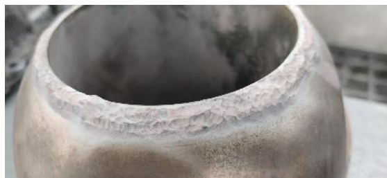
Ball Valve corrosion repair France
