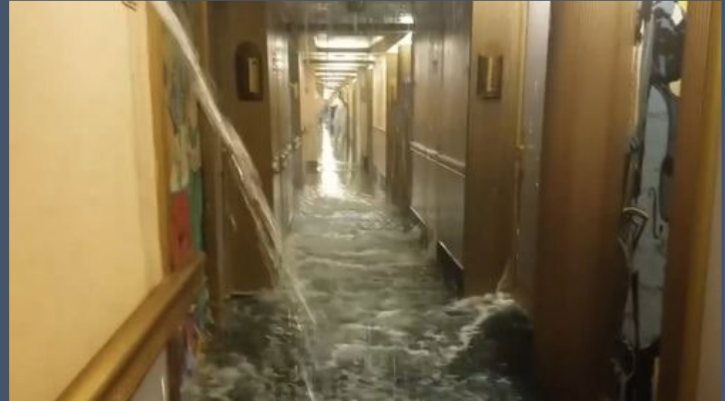
Carnival Dream fire-main discharge
