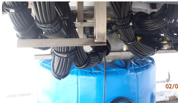
ISS HMS array in protective jacket, installed
