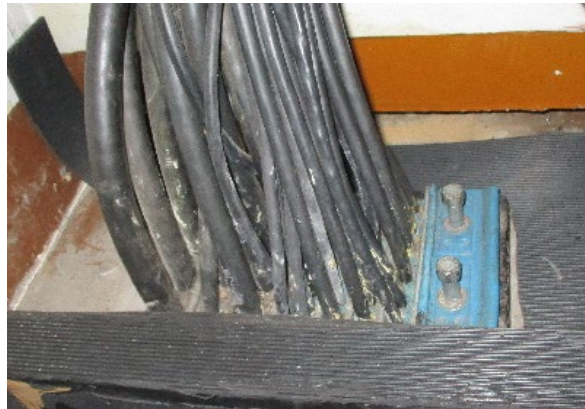
Full Roxeltec frame with 36 cables.
