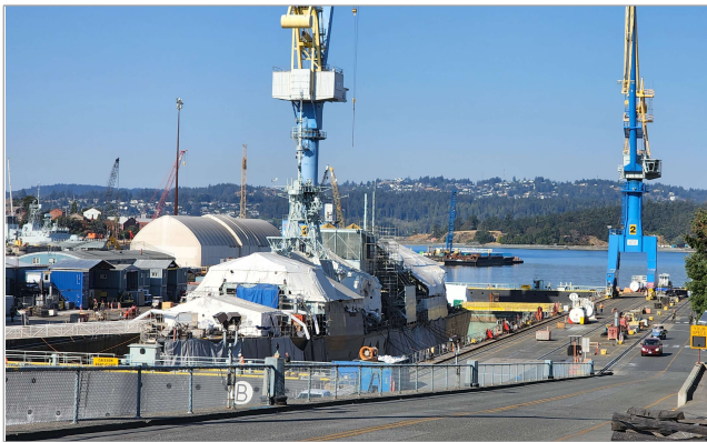
Dockyard Work Period
