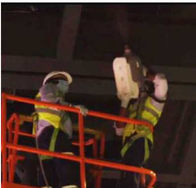
Air change rate in the halls is 8 times per hour. Air extraction in the halls is pre-scheduled and all hall shutter doors will be kept open both before and after the event to assist with air circulation
