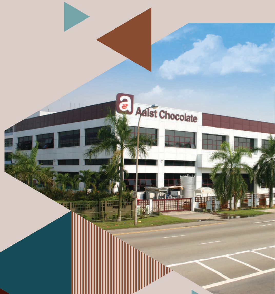
AALST CHOCOLATE MANUFACTURING PLANT Tuas (Singapore)
