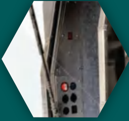
12V Electrical Control Panel
