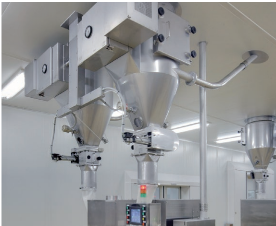
レシーバー型施工例 Example of Receiver Model installation
