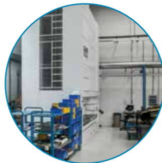
Automated warehouses and bar coding system for total material traceability
