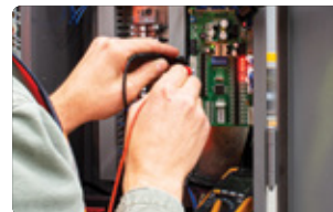
On Site Repairs
