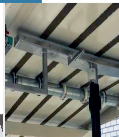
Bottom conveyor cleaning
