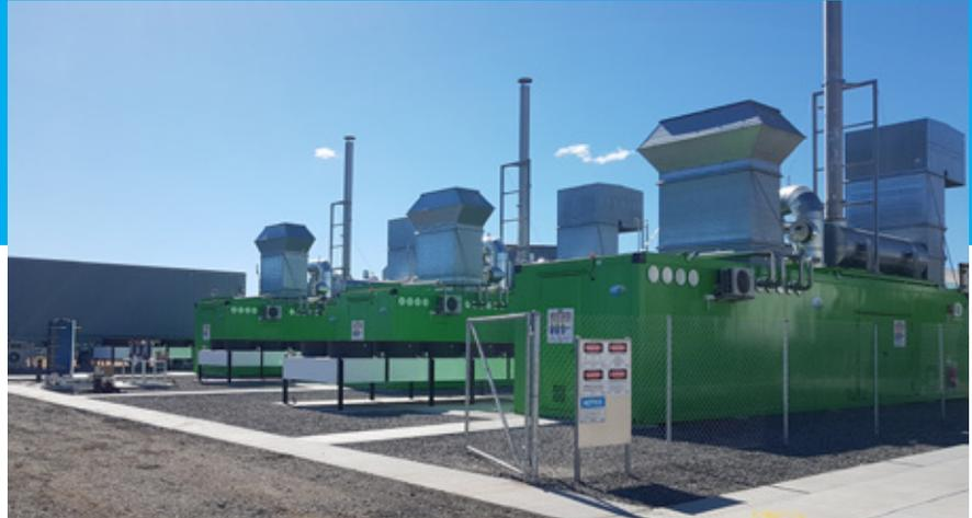
In total, 3 CHP units totalling 4000kW were installed and convert waste product to renewable energy. This project also included the supply and delivery of a turnkey biogas treatment plant including: TS biological scrubber, 2 biogas blowers, 1500kg active carbon filter tank, biogas analyser and heat pumps for scrubber temp control and gas chilling.
