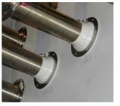
Pipetite ReBoots installed Fully flexible and capable of absorbing the pipework movement without falling away from the wall. Self sealing ribbs mean no need for use of Silicone sealants.
