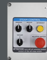
External control panel to command the belt cleaner functions
