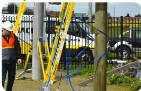
Step 6 Ascend ladder to desired position. Use work positioning hook to attach to rung hook.
