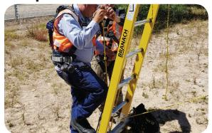
Step 5 Attach harness to the fall arrest device. Test weight on system.
