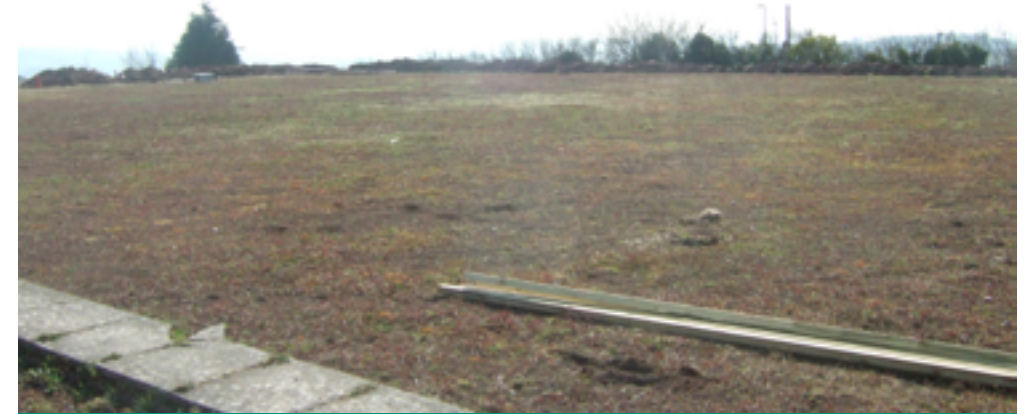
Before LINE-X Application
