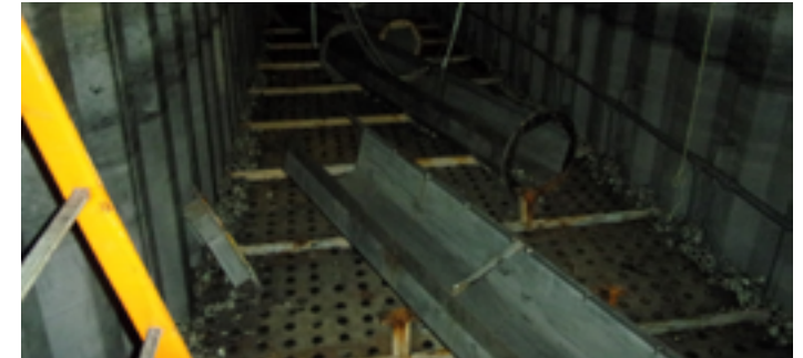
Tank prior to lining
