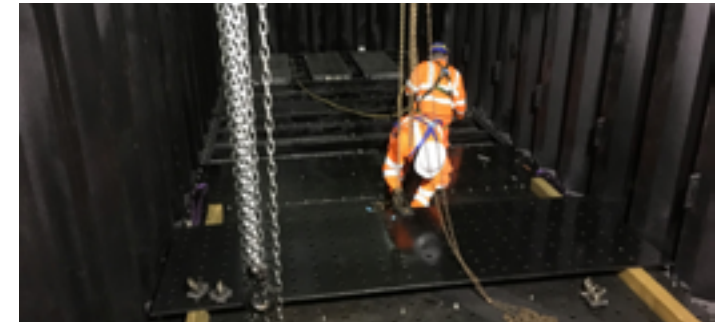
Tank during application
