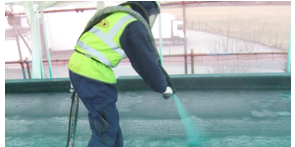
During LINE-X Application
