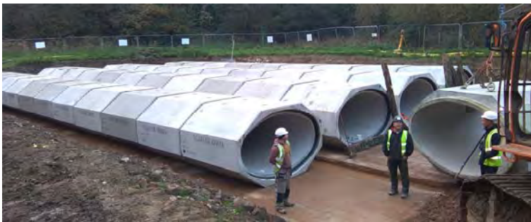
Elliptical Attenuation Tank installed at Talbot Green
