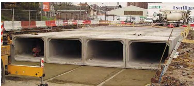
AquaCulvert with integrated dry weather flow channel used for attenuation
