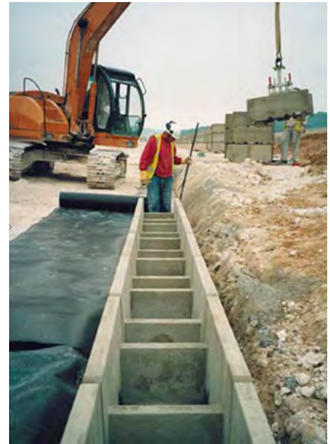
Installation on High Speed 1 for track bed sealing
