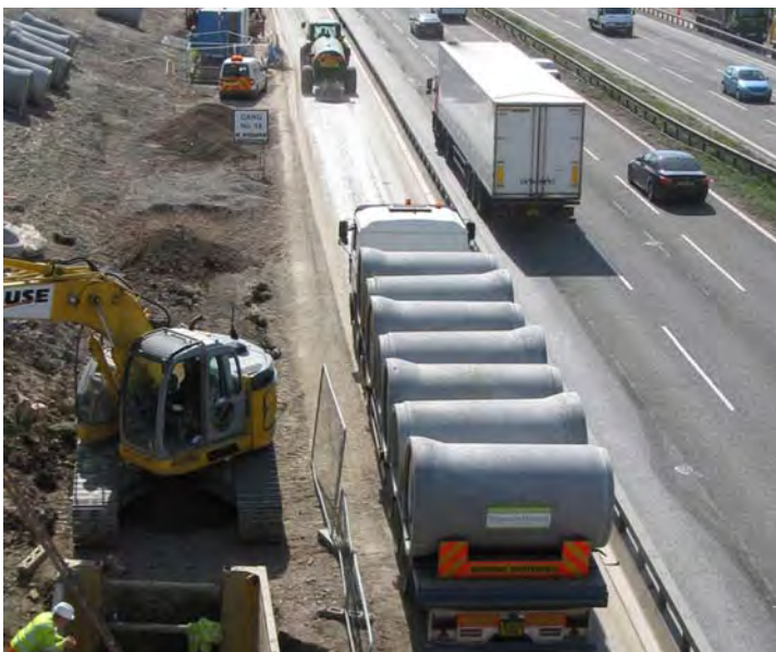
Delivery to the M1 widening scheme
