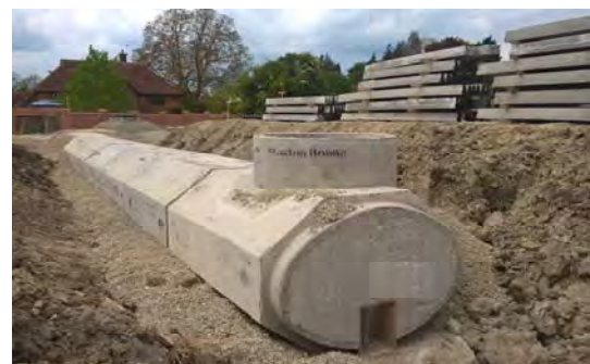
Side Entry Manhole with Elliptical Pipe
