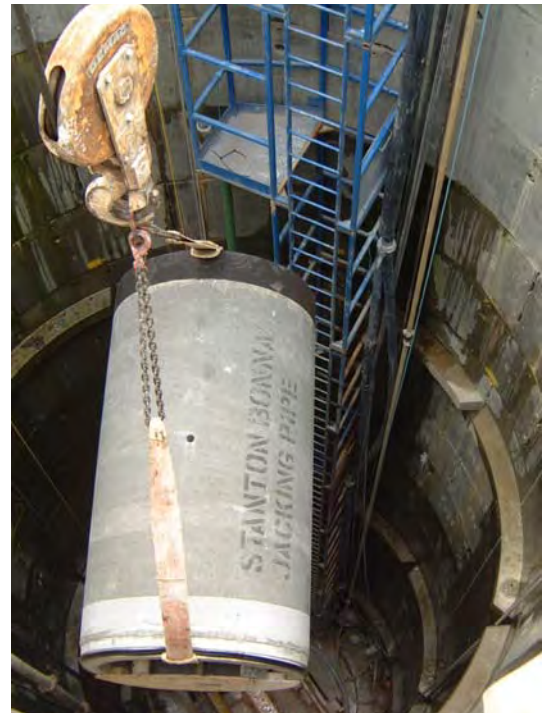
Jacking Pipe installed 26m underground
