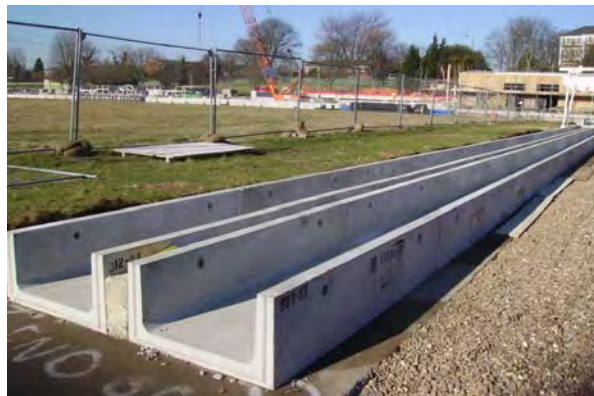
Hampton WWTW service duct installation
