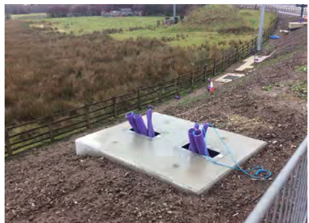
AMI Base used on Smart Motorways for M3 and M1
