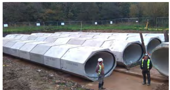
Elliptical Attenuation Tank installed at Talbot Green
