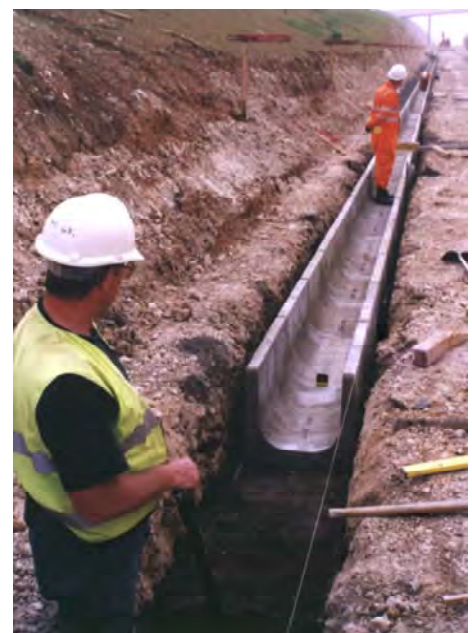
Modular components permit rapid installation
