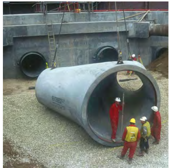
DN 3000 Y-Piece Reducing Unit
