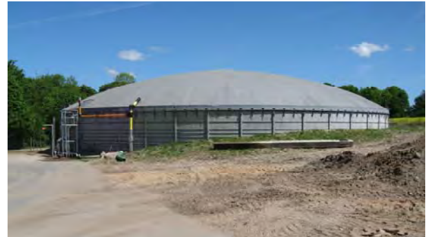
XPRES tank® used in biogas production
