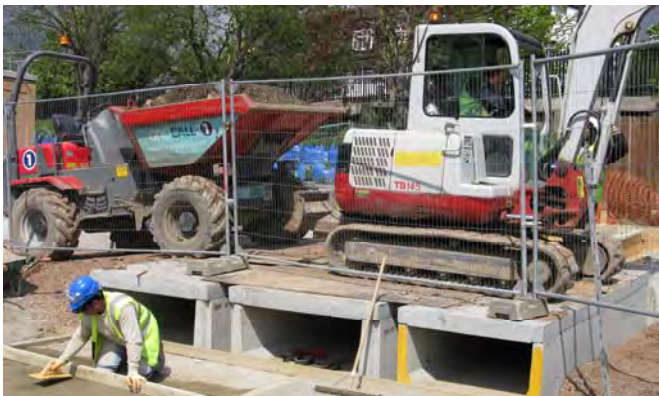
Heavy duty troughs and covers for vehicle loading
