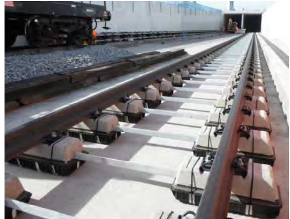
SAT S312 Twinblock Sleepers installed at Connaught Tunnel Crossrail
