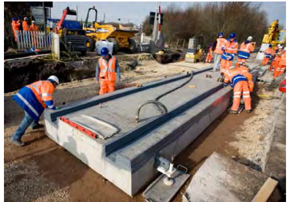
Harmelen Level Crossing installed for Network Rail
