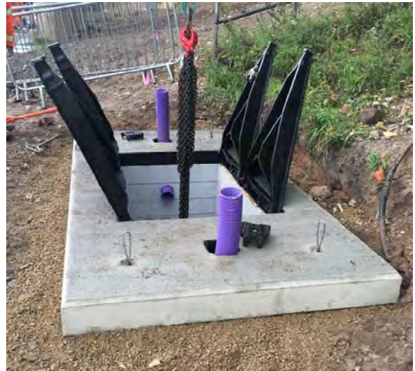
Communications Chamber Cover and Hard Standing used on Smart Motorways for Manchester and M3
