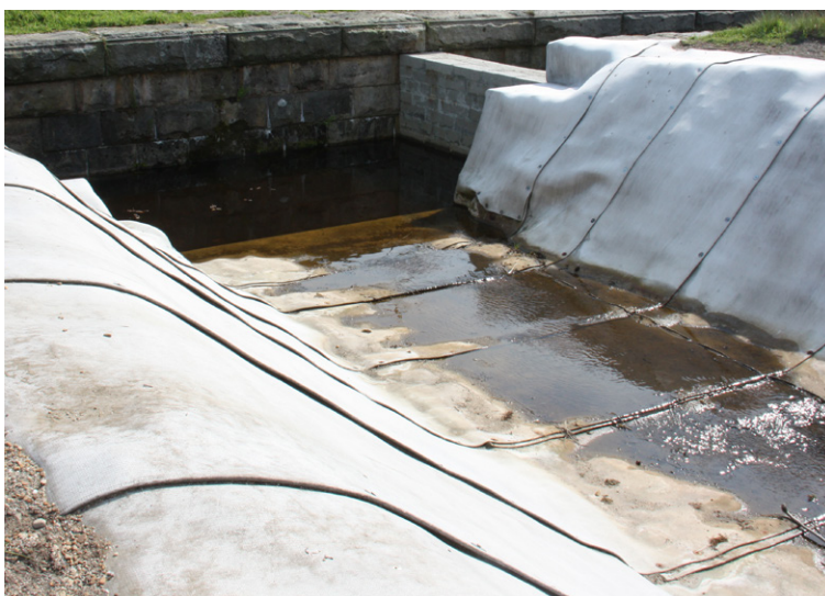
The drainage channel after hydration.
