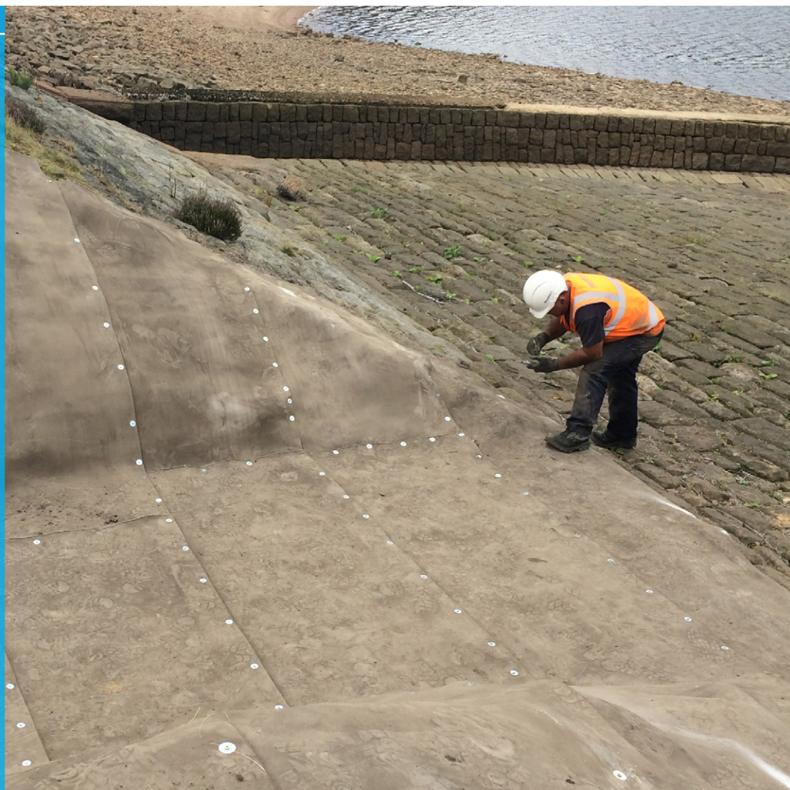
Drainage channel prior to hydration.
