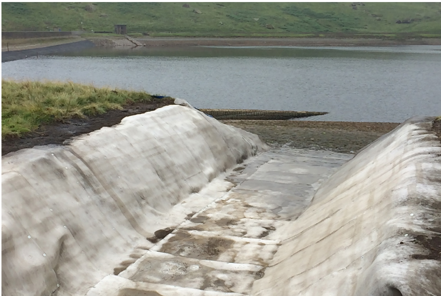
Completed drainage channel installation.
