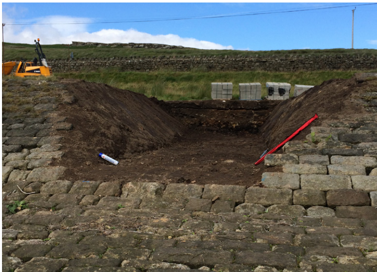
The drainage channel after being excavated.
