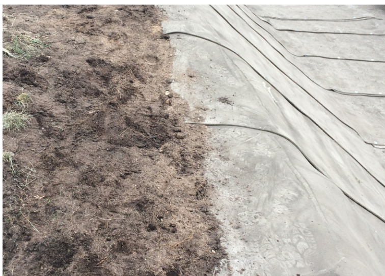
The CC was back filled into an anchor trench.
