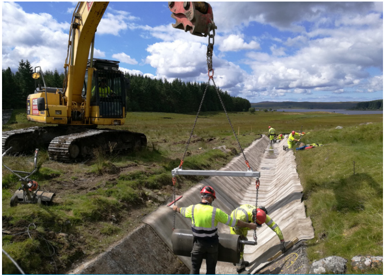
CC dispensed with a spreader beam & cut to length
