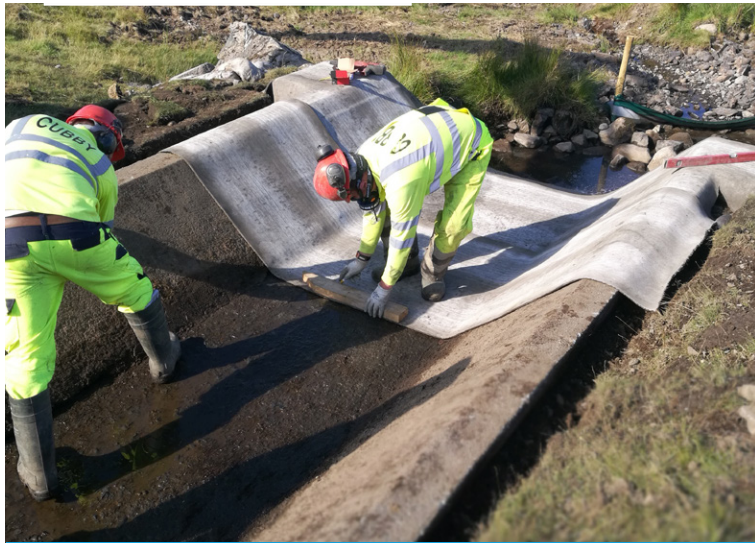
First layers of CC being laid into anchor trench & overlaps marked
