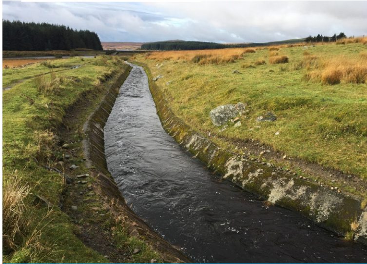
Water flow in original concrete flume
