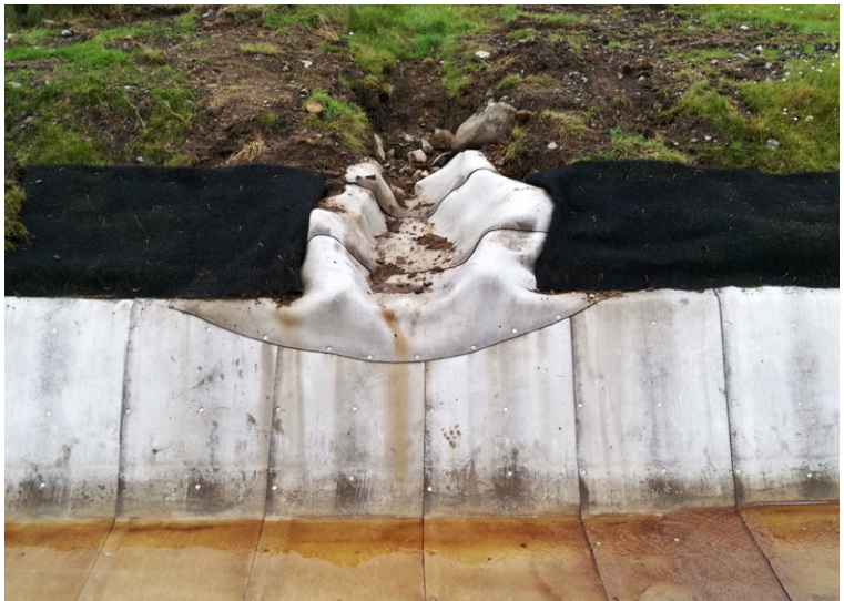
Inlet ditches lined with CC to direct bank runoff into flume
