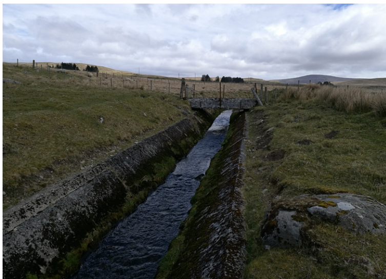
360m dilapidated concrete slabbed flume prior to installation
