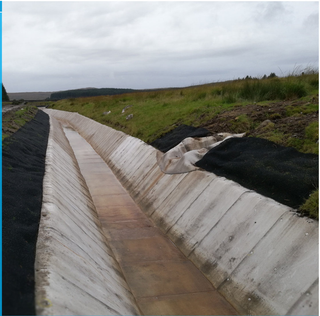
Completed installation at Muck Burn Flume
