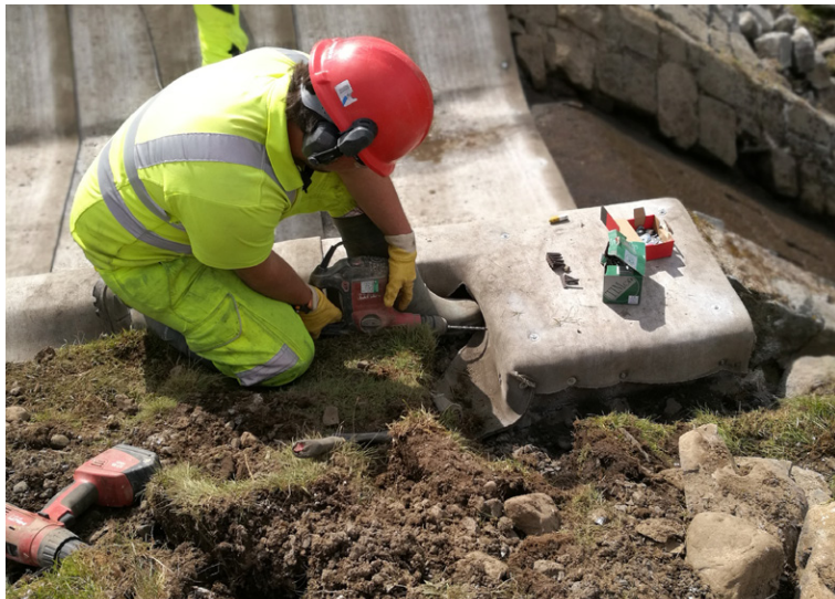
Installing 34mm Hilti nails with 25mm washers
