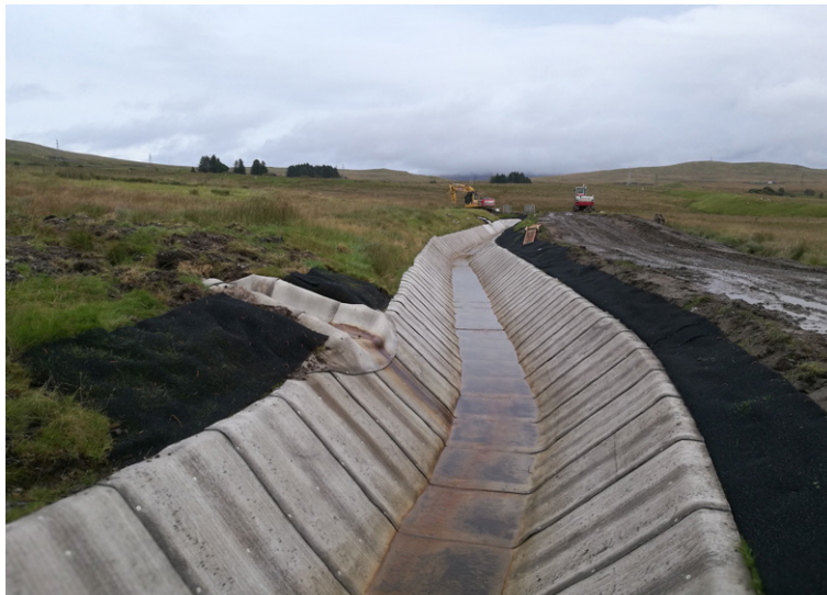
Remediated flume lined with CC8™ transverse layers
