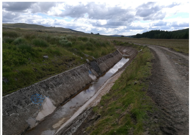
Vegetation & algae removed and water diverted out of the flume
