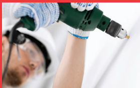
General Installation & Construction
