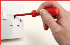
Minor Electrical Works
