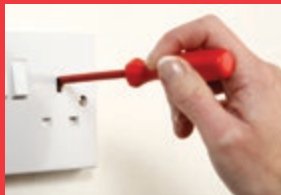
Minor Electrical Works
