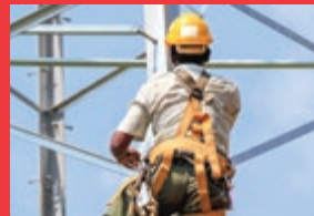
Work at Height
