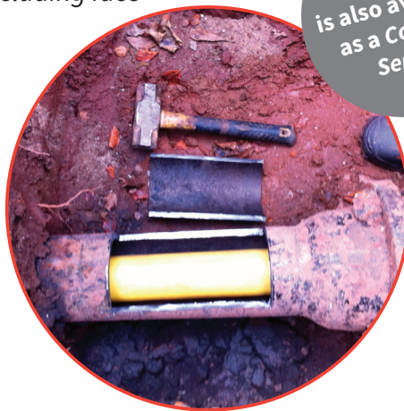
2. Window removed to reveal inserted PE
