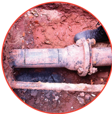
1. Circumferential and longitudinal cuts made in 100mm/4" ductile pipe
