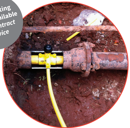
3. Service connections made to the new main
