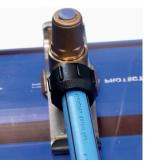
aligning the outlet to the desired position, tighten the securing collar and compression fitting and test T and connections prior to drilling.
