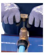
NB. You should feel growing resistance before the cutter turns easily and then stops. It is normal to get slight discharge of water during this operation.
