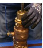
4. Attach the 110V power drill to the drill stem and apply slight pressure whilst drilling the main until there is no resistance (main wall drilled).
