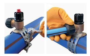
4. Fit the Protecta-Line service pipe into the compression fitting on the outlet, as described in the instructions on page 37. After aligning the outlet to the desired position, tighten the securing collar and compression fitting. Test T and connections prior to drilling.
