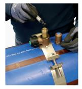
6. Ensure the cutter is fitted with the liner before installing it in the ferrule body. The cutter shall be turned down flush with the top of the body before fitting the ferrule cap. Make sure the
