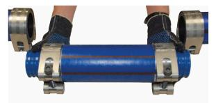
**6.** Slide the repair coupler inserts into the cut pipe ends, so all of the depth marks are visible.
