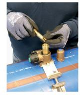
4. Make sure the small seal is placed in the cap. Replace and tighten the cap. Fit the Protecta-Line service pipe into the compression fitting on the outlet, as described in the instructions on page 37. After
