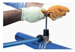
6. Withdraw the cutter all the way up to the top of the stem, employing a final counter-clockwise torque of 12-14Nm to ensure a good seal. Some leakage through the plughole is normal before the cutter has been fully unscrewed. Replace the plug.
