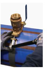
NB: For main sizes 315mm and 355mm, apply a torque of 40Nm - 44Nm.
