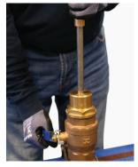
6. Position the liner insert onto the carrier of the liner insertion head. Fully withdraw the liner into the liner insert head.
