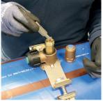
4. Fit the drill key into pre-cutter and turn down until pre-cutter comes to a stop. Once pre-cutter comes to a stop, retract it fully from the ferrule body.
