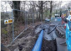
The gravel, cobble and boulder ground conditions were particularly onerous and the environmental sensitivity of the river paramount. At one stage during the works we had more ecologists on site than drillers. The bore was successfully completed to the satisfaction of the clients and overseeing authorities in an 18-day operation, with minimal impact to the river and no health and safety incidents encountered.
