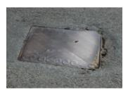
Access covers in the carriageway can become slippery over time, their raised patterns worn by decades of traffic sometimes leaving a polished slippery surface.
