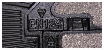
The results proved to be very encouraging with an average PSRV (polished skid resistance value) recorded of over 75, meaning only a 6% loss in performance after 12 years of continuous service, proving the long term durability of GripTop.
