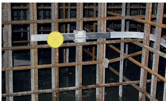
The HEA Earthing System is the universal connecting option for all earthing, potential equalisation and lightning protection components according to DIN 18014, VDE 0185-305-3, respectively EN 62305. The system offers many application variants and an extensive range of accessories for the areas of house connection, transformer station, substation, power station, signal box, bridge construction, sewage treatment plant, telecommunication.
