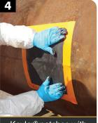
Kevlar® patches with 3X resin application (5 layers)
