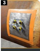
Steel plate application (with filler & magnets)
