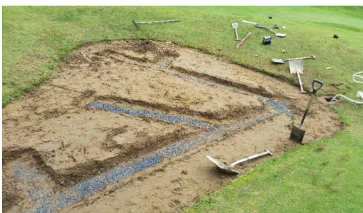
Marking out installation (10.00 am)
