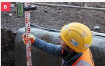
2. Position trough using cast in lifting sockets to required line and level.
