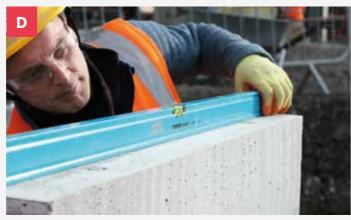
3. Position adjacent trough and, where required, apply polyurethane sealant between units.
