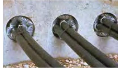
**RDSS Rayflate inflatable duct seal**
