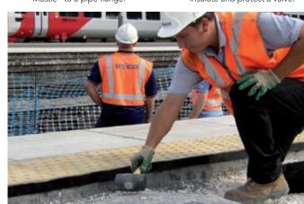
Concrete to asphalt platform joints sealed with the Denso Road System, UK.
