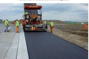
Runway re-surfacing, UK, mastic asphalt joints sealed with Denso Road System.
