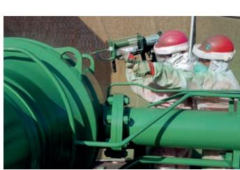
Protal 7200™ spray applied to pipeline valve in Dubai, UAE.
