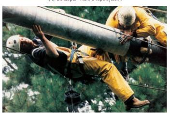
Denso Steelcoat™ System applied in-situ to protect aerial pipelines, New Zealand.
