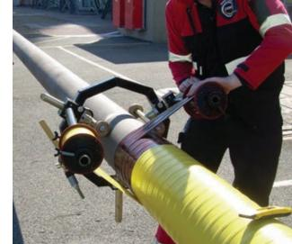
Application of two Denso tapes simultaneously using a Denso wrapping machine.
