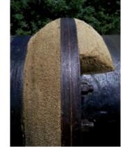
Application of Denso Profiling Mastic<sup>™</sup> to a pipe flange.
