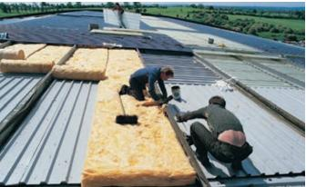
Denso Acrylic Tape prevents galvanic corrosion on 7.5 acre roof of refurbished aircraft hangar, UK.
