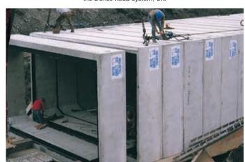
Densostrip™ Joint Sealant for precast concrete box culverts, UK.
