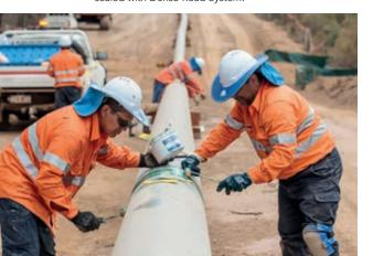
Denso™ Protal applied to Field Joints, Australia.
