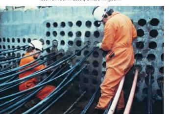
Electrical cable duct entries at UK ethylene plant, sealed with Denso Mastic.
