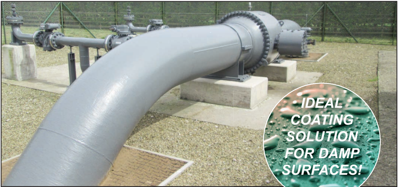
Denso Protal 7300 applied to a gas pipe.
