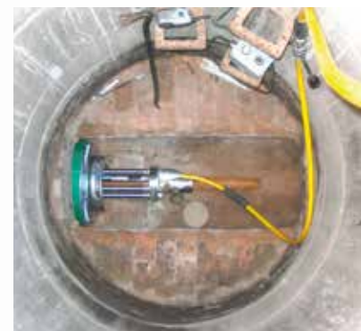
BURSTFIX 200 in the manhole
