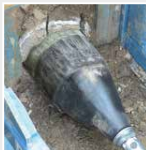
The pipe arrives at the target pit.
