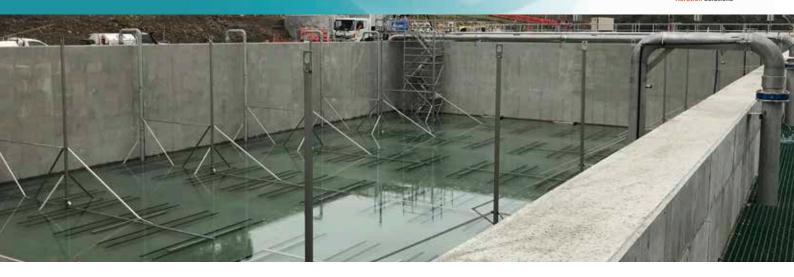
The Blackmans Bay WWTP, an Acciona / BMD Joint Venture in Tasmania, was designed with the IDEA (Intermittently Decanted Extended Aeration) process in order to enable wastewater treatment capacity beyond the year 2040, at the daily flow rate of 8,500m<sup>3</sup>/d.
