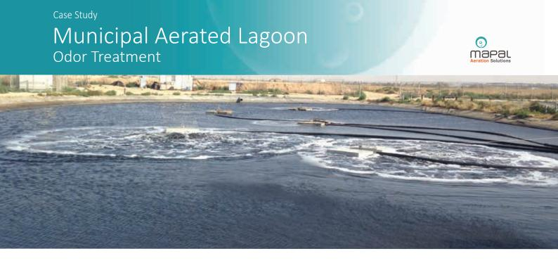
Nisgav WWTP located in the south of Israel, is operated by the local municipality and treats wastewater at an average of 10,000 m³/day for reuse in irrigation. Due to the malfunctioning exsiting aeration equipment, odors began emanating from the aerated lagoon and the municipality received numerous complaints from the neighboring residents.
