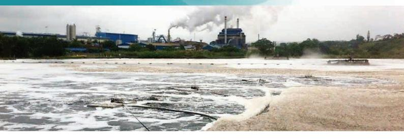
The client, a large pulp and paper mill in South Africa, produces fine paper from bagasse. The mill uses an aeration lagoon to treat the wastewater before discharging into the local river. Before Mapal's installation, the plant was using a combination of surface aerators, aspirators, and liquid  $O_2$  in order to reduce the COD as required.
