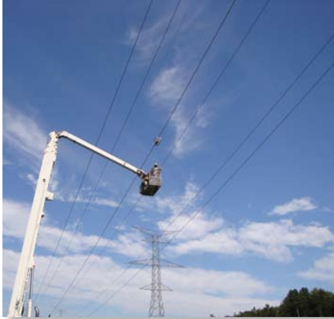
Installation from Bucket Trucks
