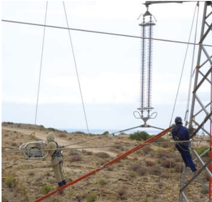
Installation from Ropes/Ladders
