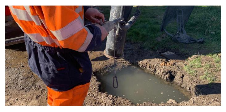
Stock Hydro-Vacuum excavators have been designed to use pressurised water to break the ground down, effectively using water to dislodge the soil, water is inherently better at cutting through hard firm clay. Wet suction machines do not require filters as water naturally suppresses dust, meaning they do not suffer from this reduced suction performance, no matter how saturated the spoil is.
