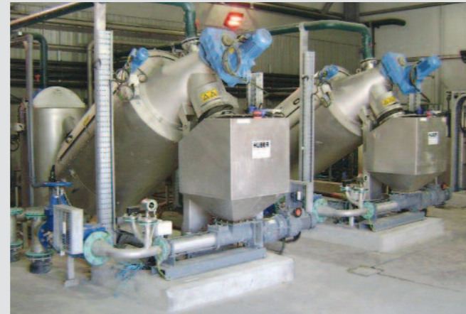
S-DRUM installation at Enniskillen
