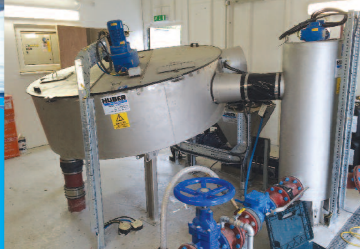
S-DISC installation at Welshpool STW
