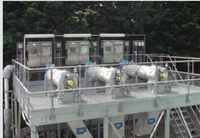
STRAINPRESS® installation at Riverside STW
