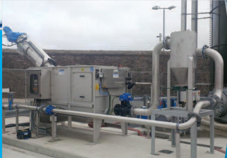
Ro3 installation at Pembroke Dock
