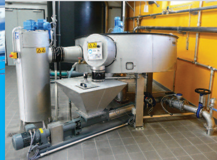
S-Disc installation Compact, enclosed sludge thickening
