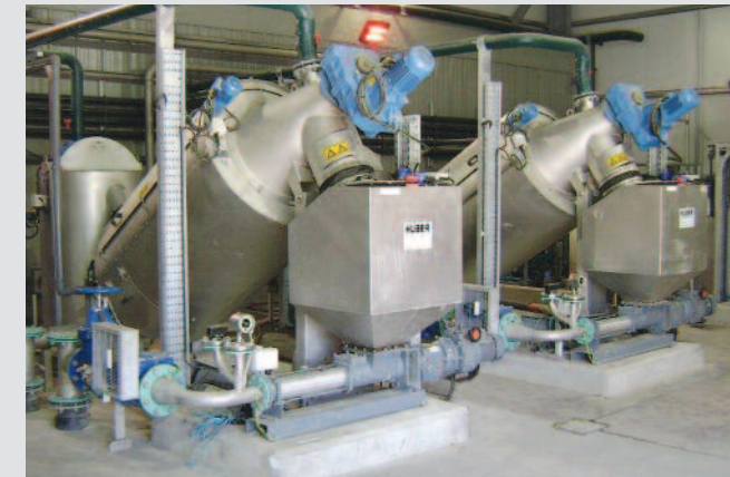
Multiple units installed in parallel for larger flows
