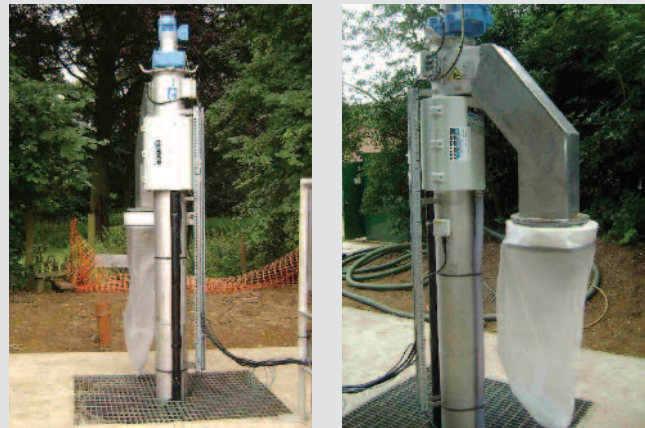
RoK4 installation discharging screenings directly into bin, with integrated bagging unit.
