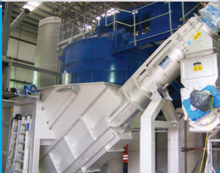
Light Fraction Screen at Bredbury Parkway
