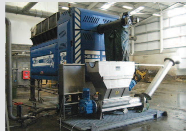
Wash Press washing and compacting reject material at Tamar
