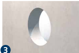
3 Core drill holes in new and existing buildings
