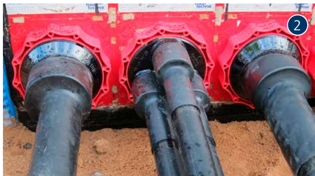
system cover HSI150 D1 and D3 – hot shrink-fit method
