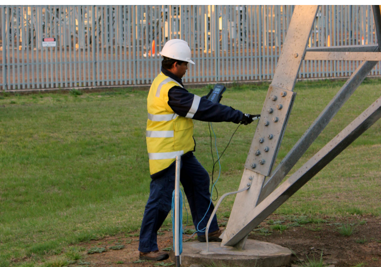
Measuring touch voltages during an injection test with the Safearth MI1 Tuneable Voltmeter
