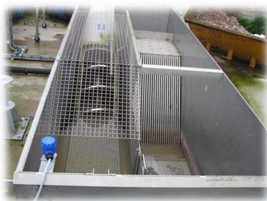
Bespoke tank design to incorporate bypass
