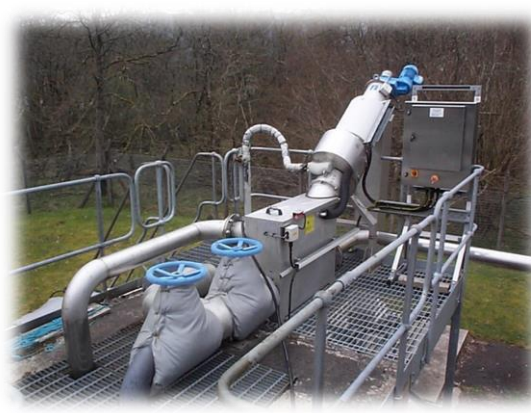
Screen and control panel installed by Huber
