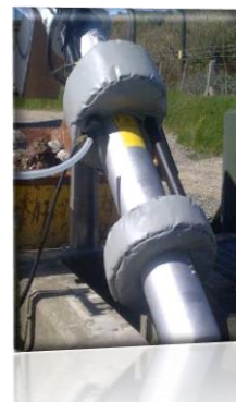
External view of ISW with frost protection
