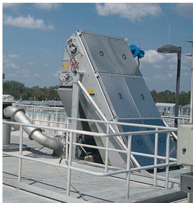
Fully enclosed, odour-free screen with easy to remove covers
