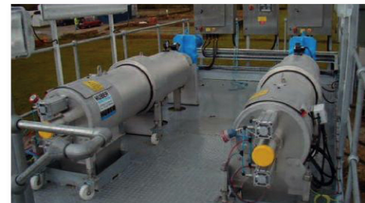
STRAINPRESS® with heatable casing pipe
