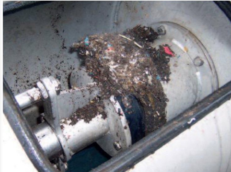
Discharge of the separated dewatered material
