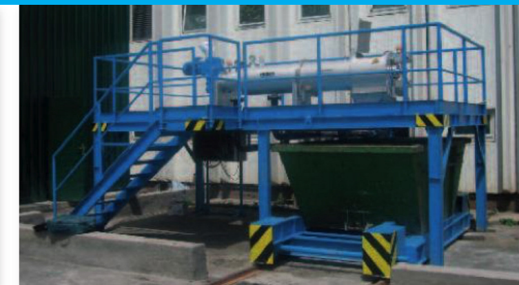
Outdoor installation of a HUBER Sludgecleaner STRAINPRESS®
